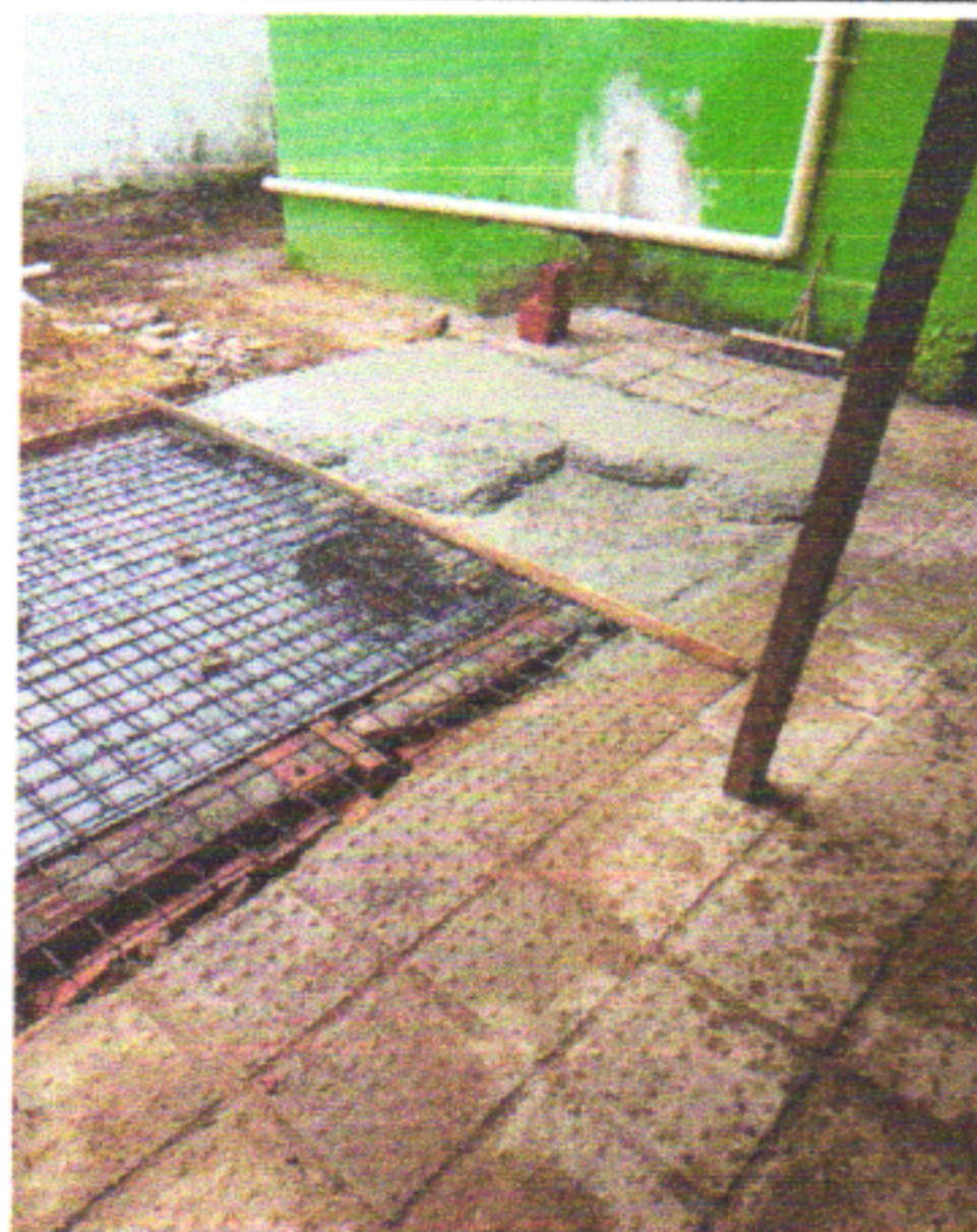
TAMPA - CONCRETO FCK = 20MPA
